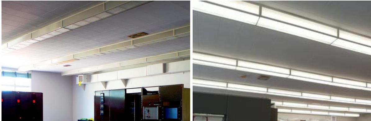
Figure 70. Original light fixtures (left) in the Oregon City Control House converted to LED lights (right).
