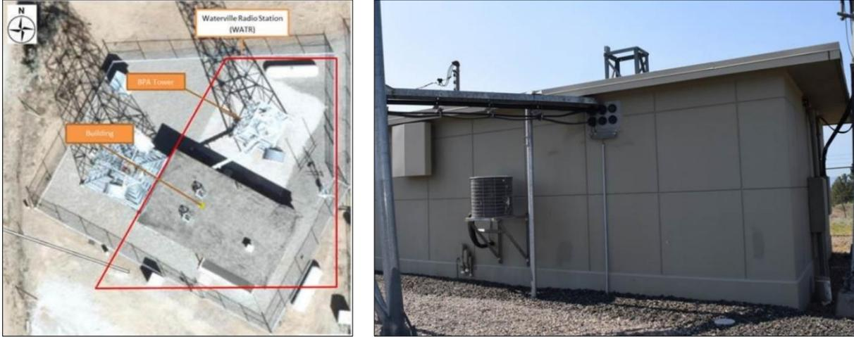
Figure 18. Penetration of the north wall of the Waterville Station Building to bond the ground bar to the outside grounding.
