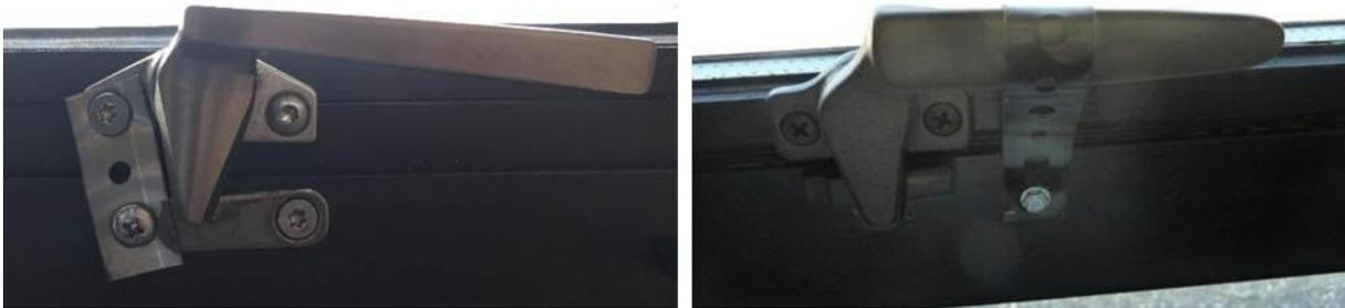
Figure 51. Non-obtrusive window modifications that inhibit operability without diminishing integrity
