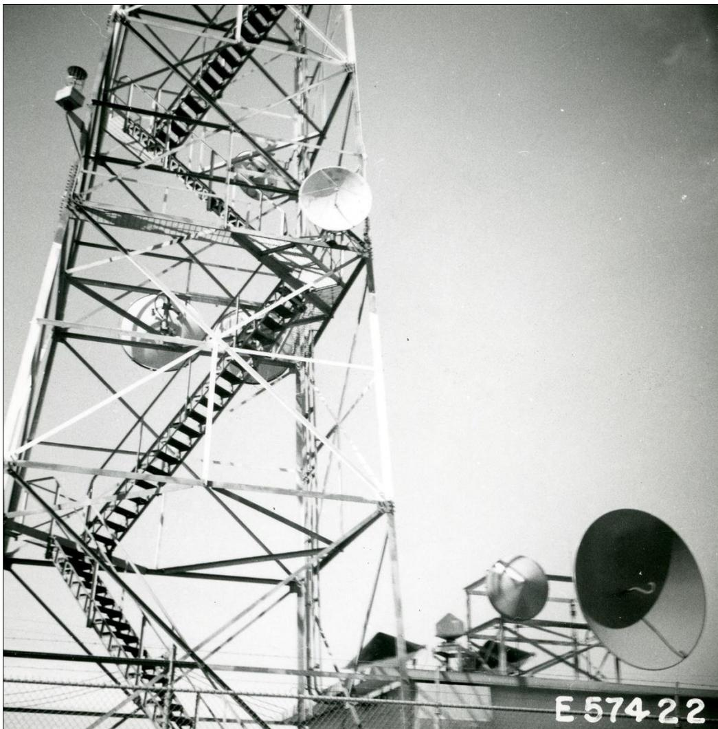
**Figure 13. Four-leg Steel Lattice Tower with Internal Staircase at Beverly Microwave Radio Station, nd. (NARA:BeverlyMWNARAbbox10-013).**
