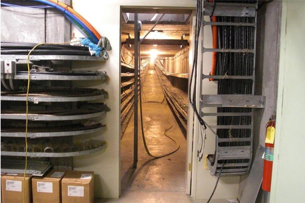
Figure 40. Boundary Substation Control House basement cable room and entrance to cable tunnel
