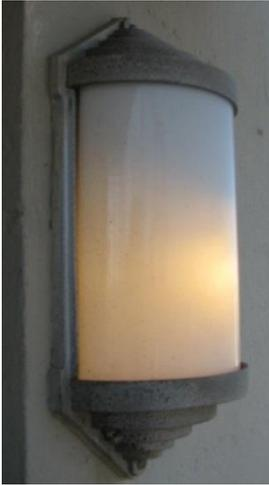
**Figure 58 Streamline Moderne-Style Light Fixture, Roundup Control House**
