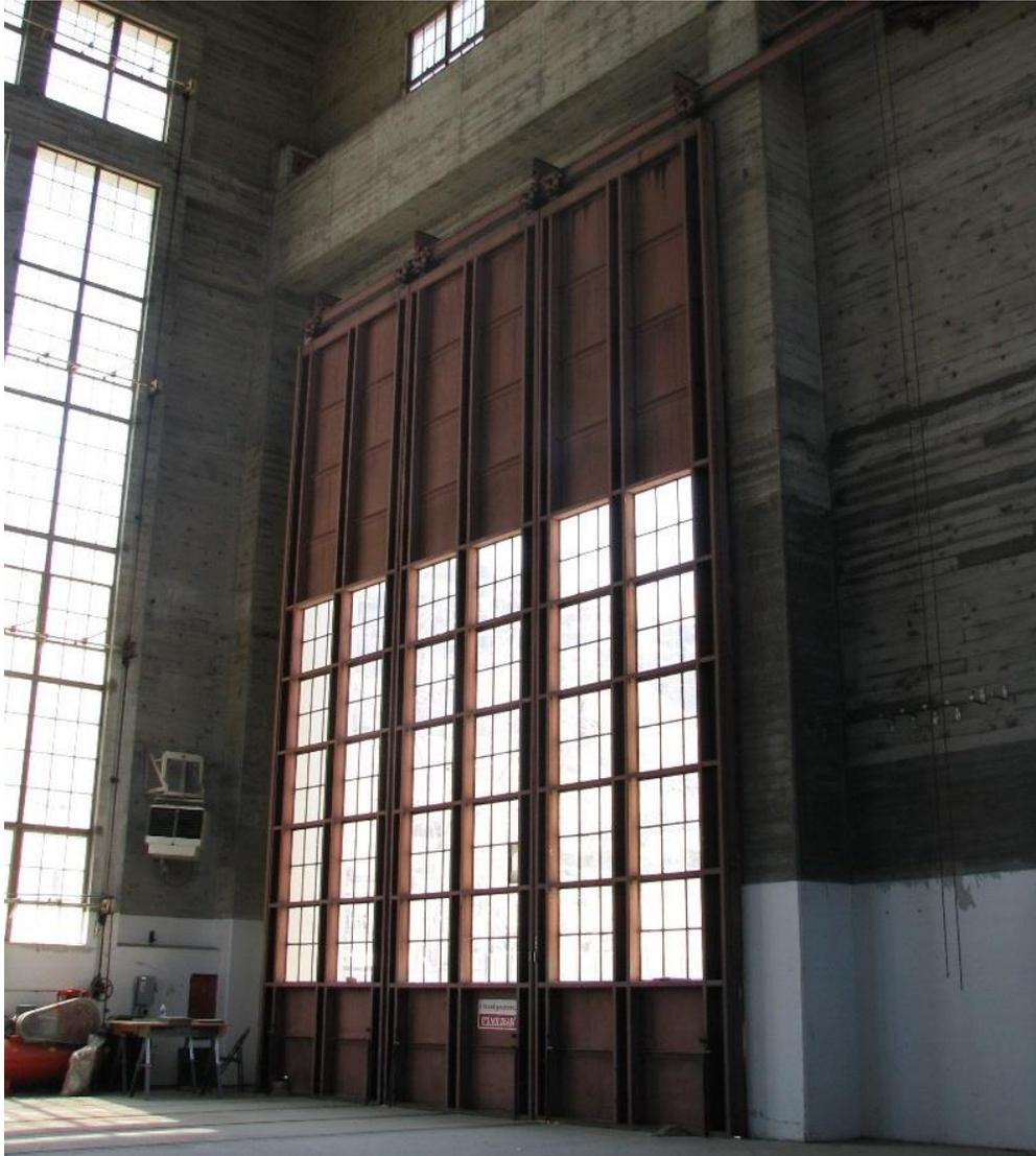
Figure 47. Untanking Tower Door, Midway Substation
