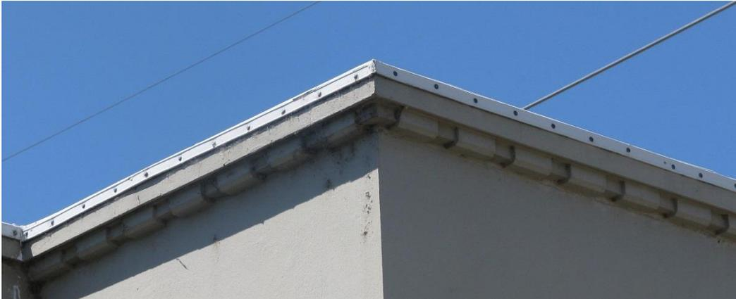
**Figure 56. Midway Control House Dentils Detail**
