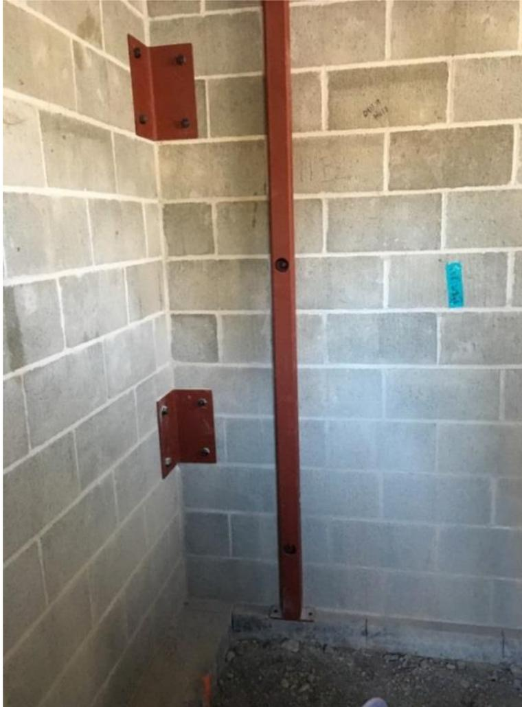
**Figure 63. Steel frame structural retrofit on building interior (Troutdale Control House Seismic Upgrade Option C)**
