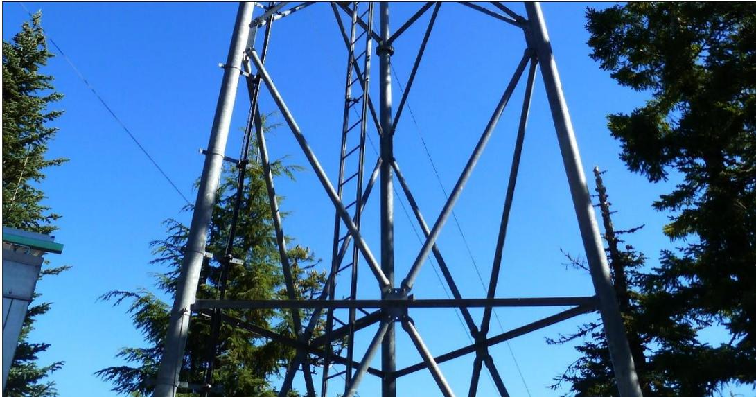
Figure 12. Three-leg Steel Lattice tower at Hall Ridge Microwave Radio Station.
