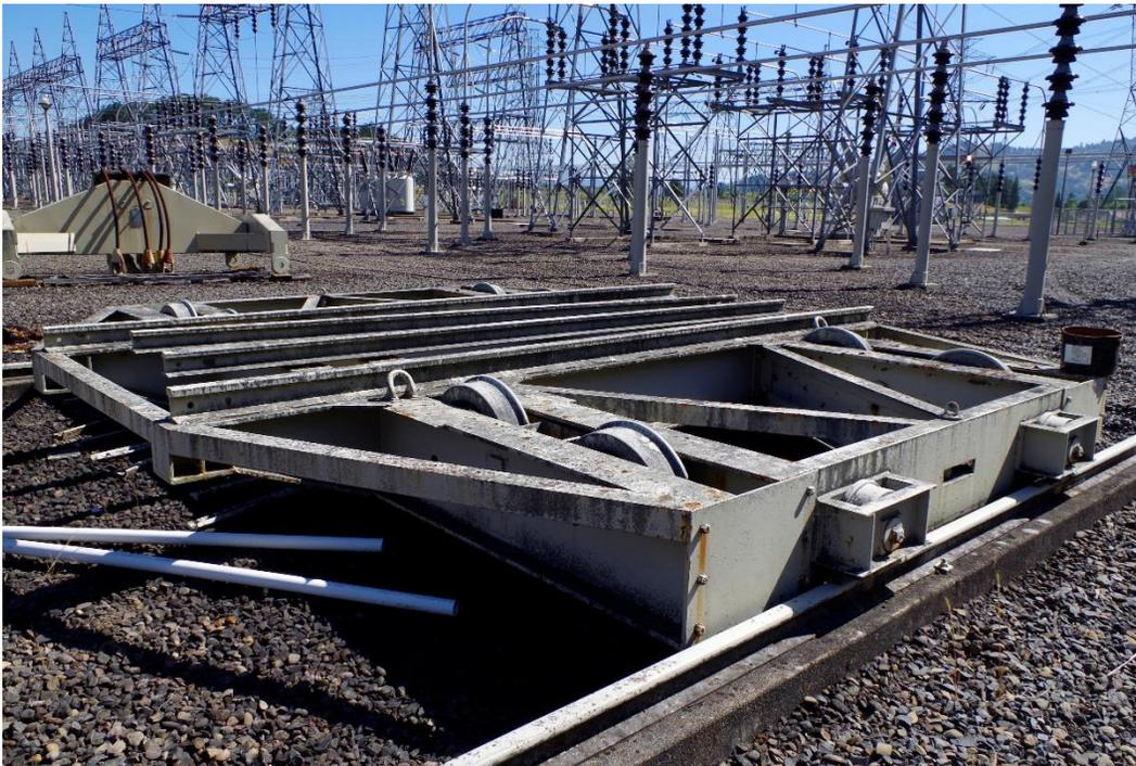
**Figure 39. Alvey Substation Transfer Cart and Rails**
