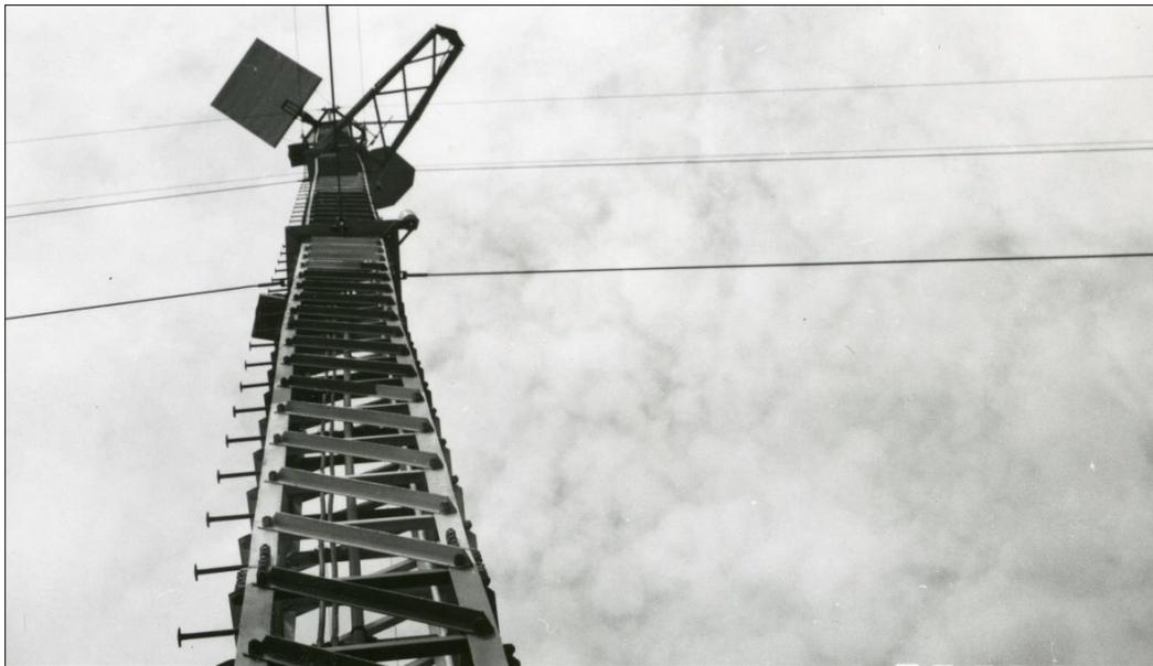
**Figure 14. Four-leg steel Lattice Tower with Guyed Wires at Leneve Microwave Radio Station, 1961 (NARA:LeneveNARAbbox15of52-003).**
