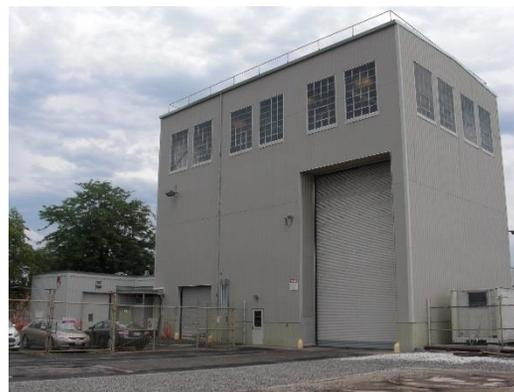
Figure 48. The Midway Untanking Tower with its original distinctive door retains overall integrity, while the new roll-up door diminishes the integrity of the Bell Untanking Tower.
