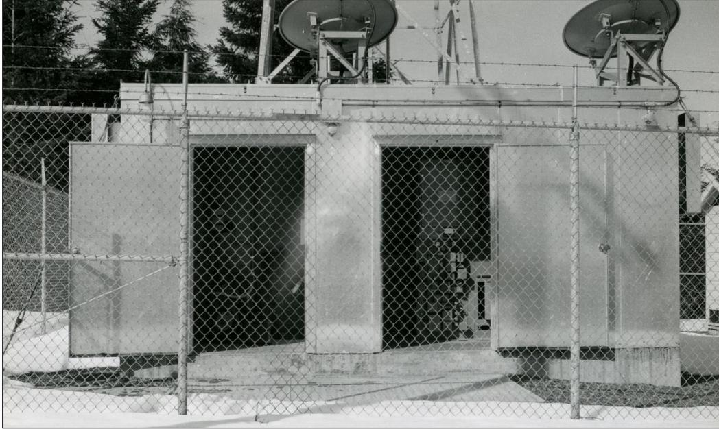
**Figure 9. Type 1503 Noti Microwave Radio Station Building with Engine Generator Room on Left and Radio Room on Right, 1956 (NARA:NotiMWNARAbbox19of52-008).**
