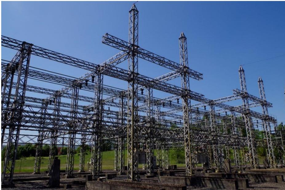
**Figure 16. St. Johns Substation Switchyard with Lattice Superstructure**
